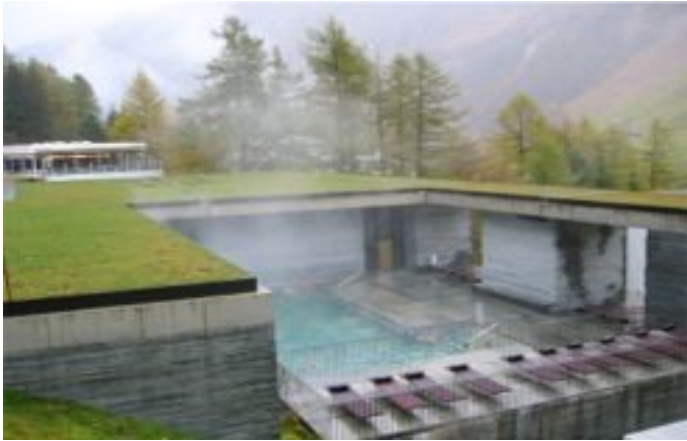
Architect Peter Zumthor's naturalistic approach in the Swiss Alps.
