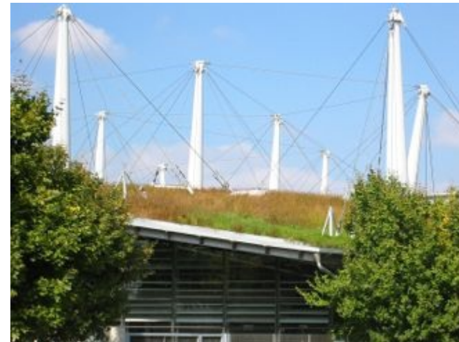
The world's only suspended greenroof in Lyon, France; Photos by Haven Kiers
